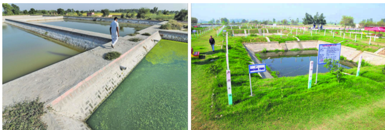
Figure 27: Photograph depicting Waste Stabilization Pond
