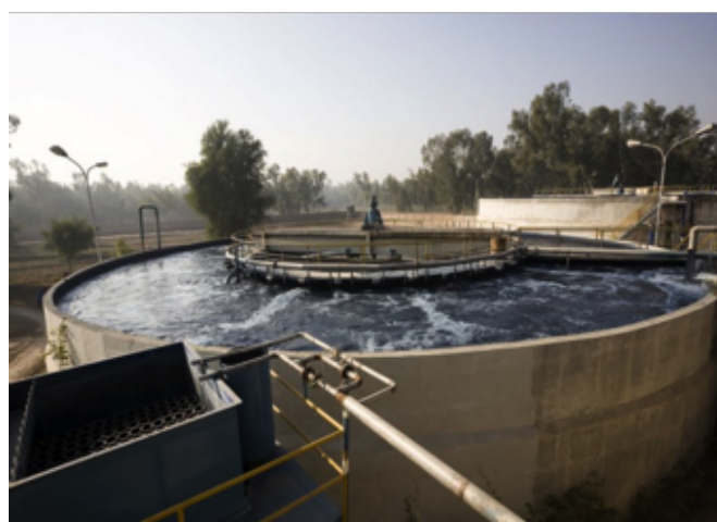
Figure 29: Photograph of Activated Sludge Process Plant
